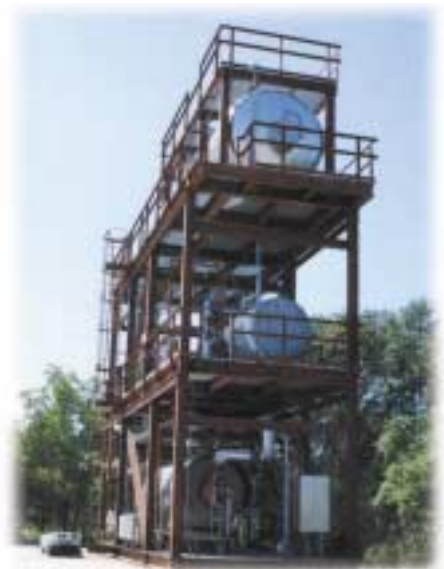
Feedwater heater skid for modular plant design.
